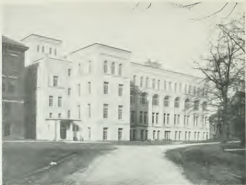
THE ELECTRICAL BUILDING
